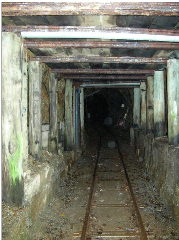
Fig. 16: Deep Adit, new railway
