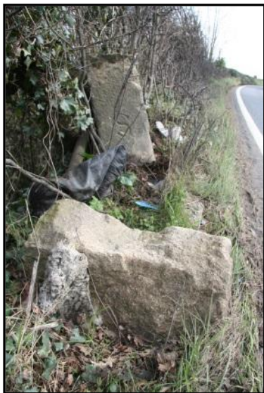
Fig.12. Milestone marking '3 miles to Saltash (Ferry)' on the Callington Road No.3 ('III mile To S') lies very badly damaged, dangerously close to, and on a bend of the A388 road, along which vehicles drive at speed. This milestone has been damaged three times and repaired twice in recent years.
