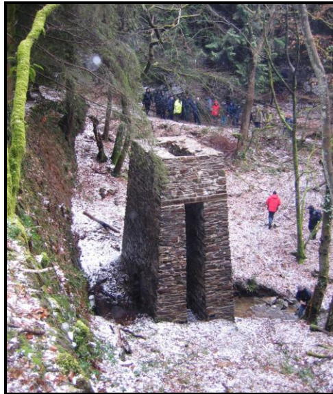
Tower of former flat rod system, Rubbytown Bottom
