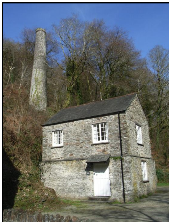
Fig.4 Engine House and chimney, Danescombe Valley
