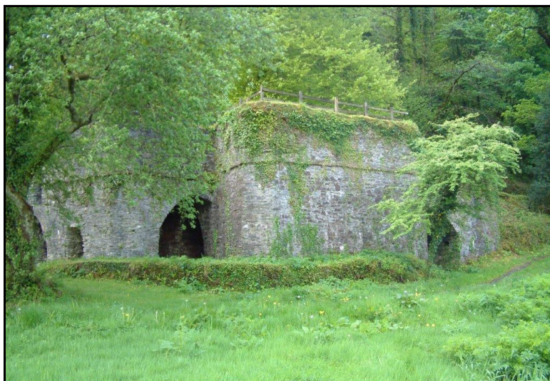
Fig. 6 Bohetherick Wood lime kilns
