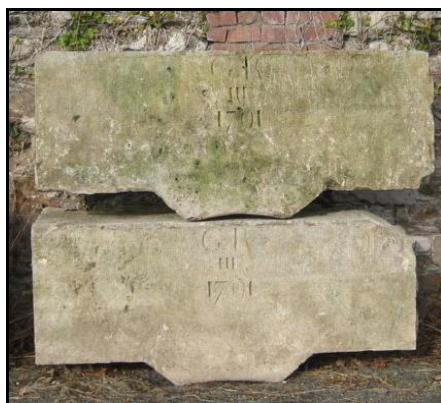
Fig.5 1791 date stones, indicating a major building phase
