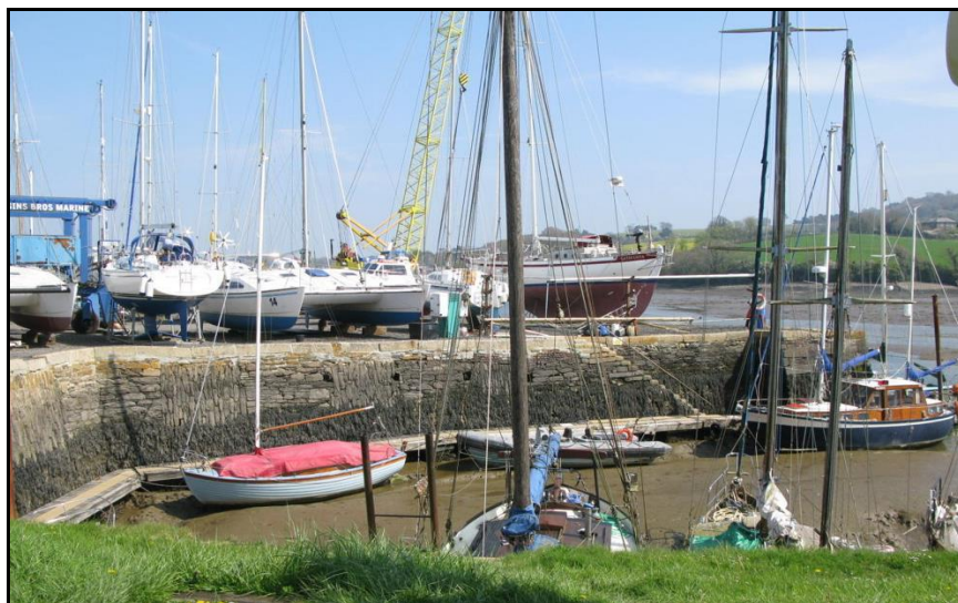
Fig.7 Southdown Quay walls April 2017
