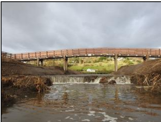
Fig.4 The new bridge viewed from the Tamar. The scale of the bridge is very evident (all photos: Pete Thompson)
