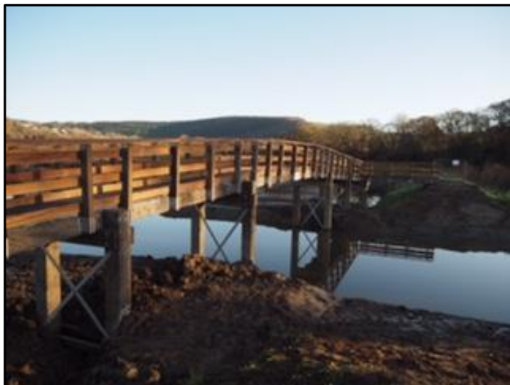
Fig.2 The completed bridge, Calstock Wetlands.
