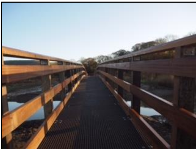
Fig.3 The bridge viewed from the walkway.
