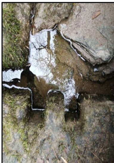
Fig. 3b. Cut slots – part of a sluice mechanism.
