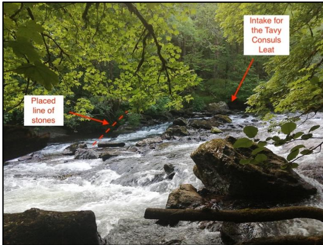
Fig. 6 Boulders across the river at the Abbot's Weir site including a line of placed stones. Also labelled is the intake for the Tavy Consuls leat.
