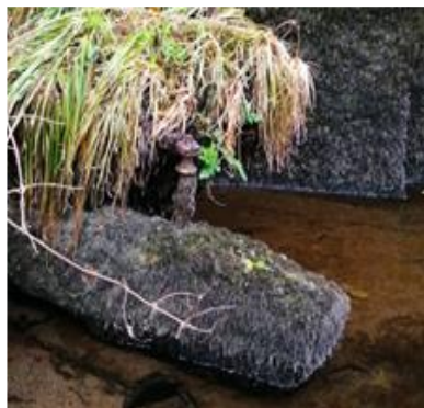
Fig.3d. Metalwork protruding from a recumbent post lying in the sluice
