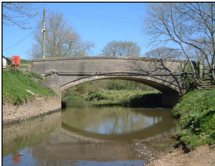
Bridge over Tamar at Bridgerule. Here, the Tamar is wholly in Devon.
