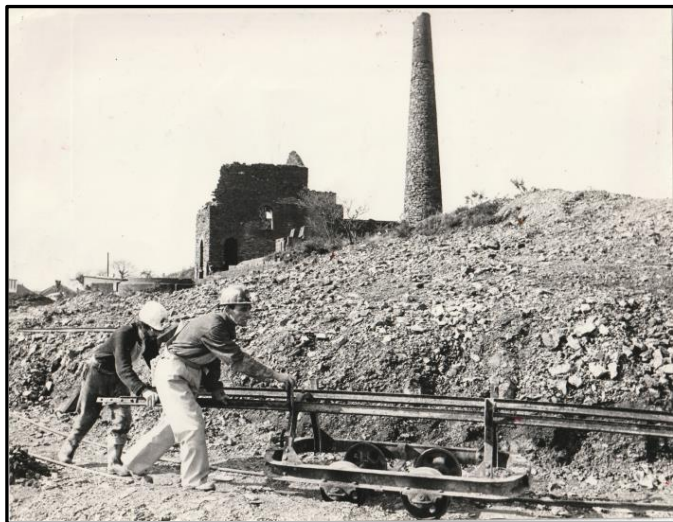
Fig.3 Pop Courtis and Alex Friendship moving rails into the new working at Prince of Wales Mine, early 1970s (author’s photo)
